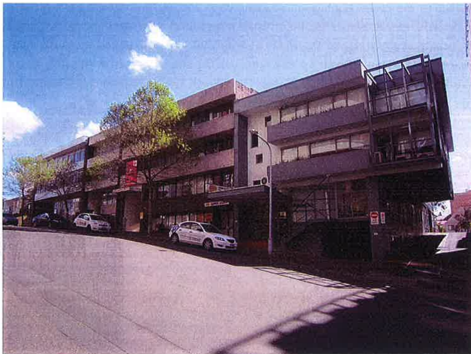
View of 18 Berry Street (right) and development adjoining the site to the west
