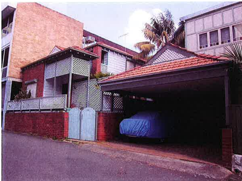
View of 1A Doohat (left) and the rear of 1 Doohat Ave (right)
